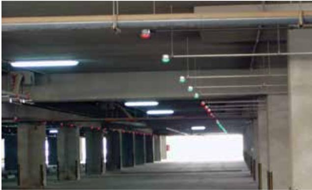
Dat - Con has developed control system, which allows a complete overview of the occupancy of parking lots and management occupancy statistics, which is by the security most important. The entire system is based on a close reading of the current situation in parking garage for determining the occupancy of parking spaces by using ultrasonic sensors. The sensors contain high lighting LED indication, which allows the user an easy overview utilization of individual parking places.
